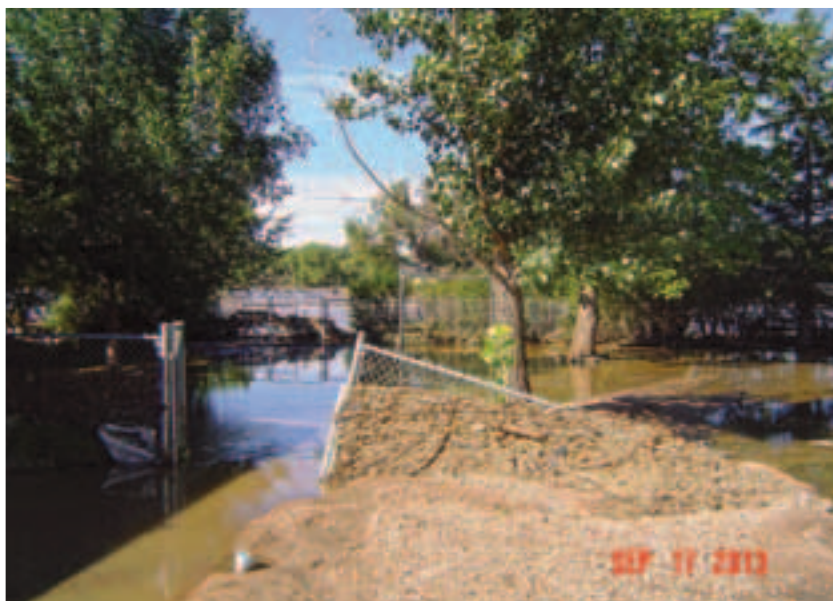
Muddied, rushing water washed out the ground from under a chain-link fence that enclosed Art Parker's yard.
