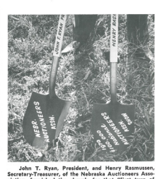
John T. Ryan, President, and Henry Rasmussen, Secretary-Treasurer, of the Nebraska Auctioneers Association, furnish the shovels for that "first turn of earth." (Lower picture) The shovels will be permanently stored in the new building.
